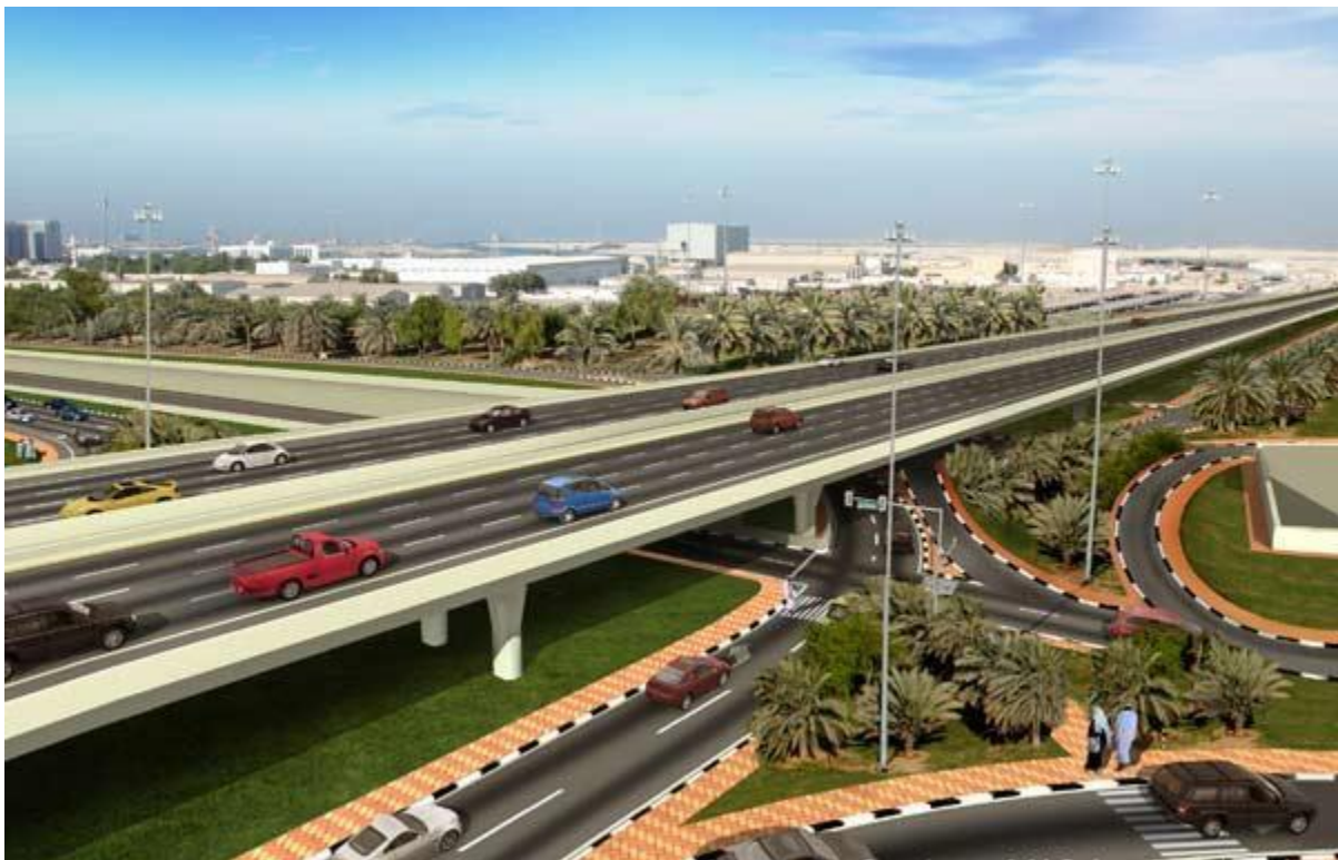
Figure (mm) Al Salam Street Project Abu Dhabi
